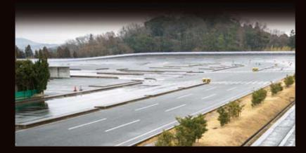
In the premises of Alpine's Head Office in Iwaki, we have an oval course that looks like a race circuit. Using this course, we drive automobiles at high speeds to investigate how the generated vibration and noise affect the navigation system and the audio equipment.
